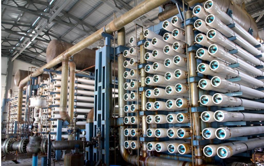
20 MLD DESAL RO Plant
